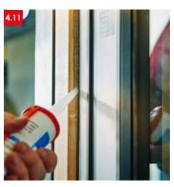
Seal perimeter with proprietary sealant. Be sure to follow sealant manufacturers instructions regarding backer rod and primer.
