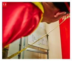
Check the opening for squareness by measuring the diagonals and check the frame for any damage.
