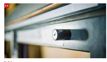
Check that the traffic door magnets have been fitted and that they align when in the open position.
