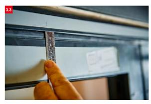
3.3 Ensure that there is a 12mm gap top and bottom between the outer frame and the door panel.
