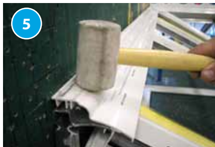
5 The PVCu wallplate top cap is exactly half of a ridge top cap and is fastened in the same manner.
