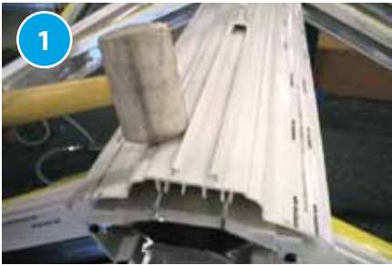
1 Centralise the two clips on the ridge top cap with the two barbs on the main ridge.
