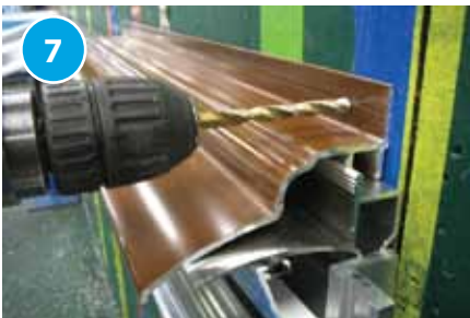
7 An extrusion line has been incorporated along the back upstand of the aluminium wallplate top cap for the positioning of the fixing screws.
