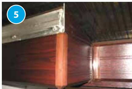
Extra box gutter under clad is supplied to cloak of the remaining raised leg section.
